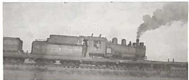
Locomotive used in laying track.
