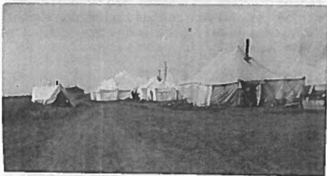
Construction camp at C.N.R. dam.
