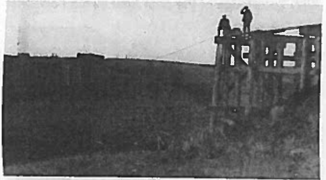
Third C.N.R. bridge under construction, 1925.
